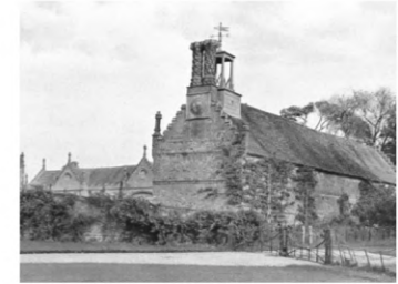
South East Elevation, Clocktower 1924
