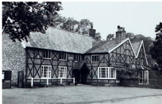
1939 photograph of the Griffin, showing rebuilt south gable and straightened roof pitch of the range on the front of the building (England's Places)
