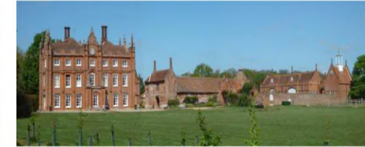
East Elevation, Cockfield Hall 2005
