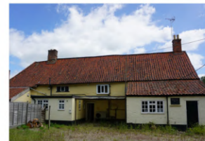
Rear elevation with 20 th Century extensions
