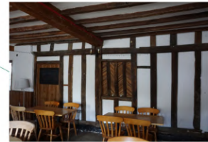
Southern room on the ground floor with early 16 th Century timber frame and later alterations
