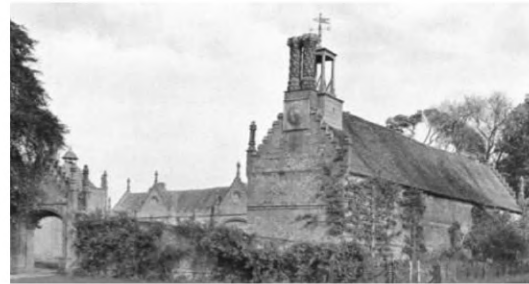
South East Elevation, Clocktower 1924
